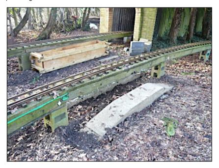
The Raised Track is now closed until further notice, whilst we make and pour concrete into the shuttering to make the four step-over blocks to assist access to the tunnel shed and the COSH cabinet.
